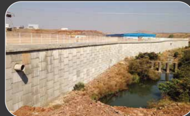
KSH Logistics & Park, Chakan, Maharashtra
