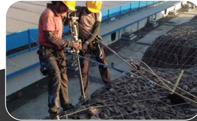
Drilling with Jack Hammer, Chakan MIDC, MAHARASTRA
