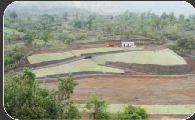
Landscaping work for Resort Project at Karjat
