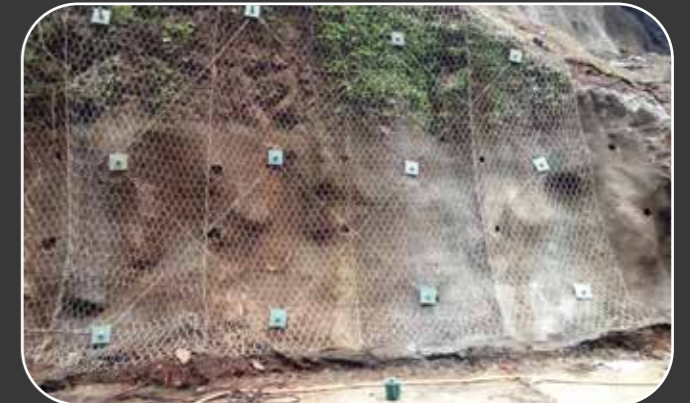
Shotcreting at Nahar Amrit Shakti, Powai, Mumbai
