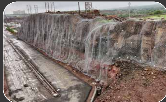
KSH Logistics & Park, MIDC, Chakan
