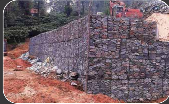
Road Embankment Retention work, for Karnataka State Highway at Madikeri
