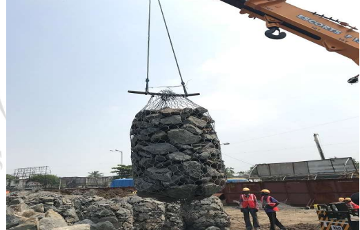
Fig:04. Lifting Prefilled Sack Gabion.
