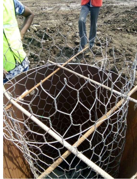
Fig:04.Arrangement to fill Sack Gabion.
