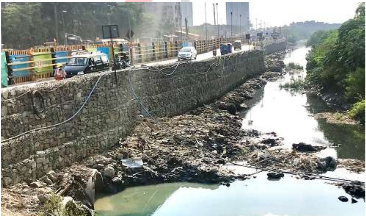
Fig:09. Completed Structure
