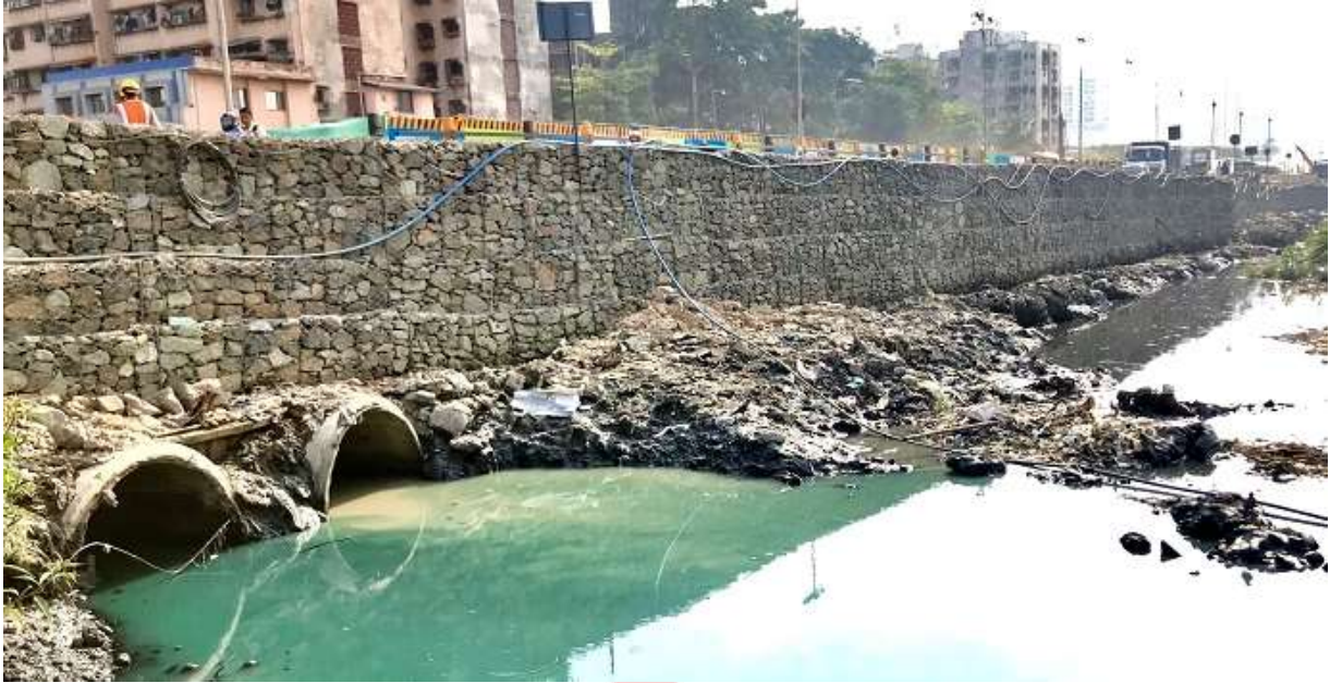
Fig:08. Completed Structure
