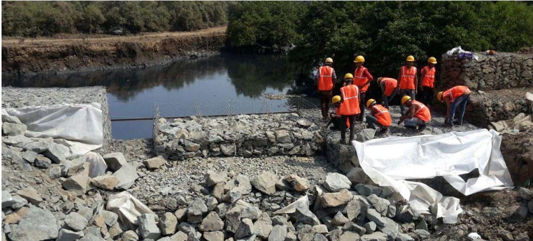
Fig:07. Filling of Gabion Boxes Over Prepared Sack Gabion Bed
