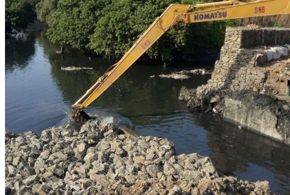
Fig:06. Launching of Sack Gabions.
