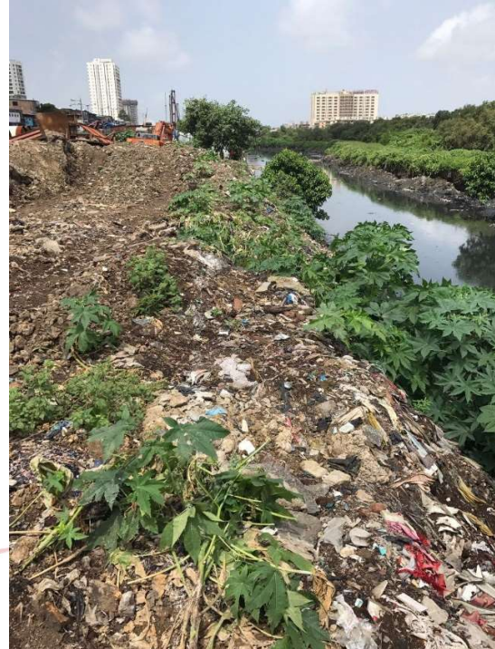
Fig:02.Before commencement of work
