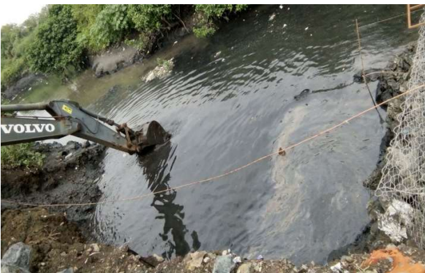
Fig:05. Excavation and removing of sludge uptil hard strata.
