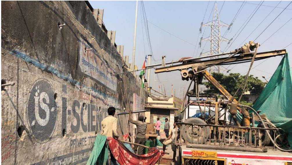
Site Photograph-Drilling 5m Deep of 75mm Dia Hole.
