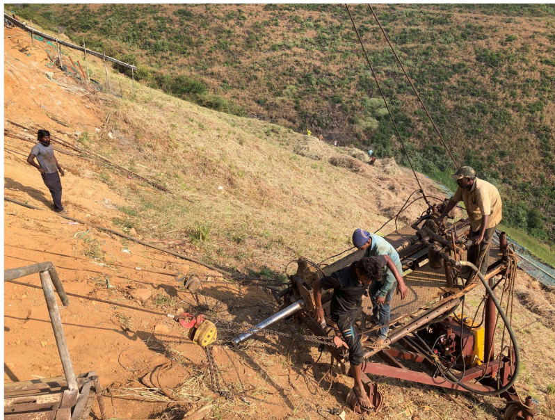
DRILLING AT 15° INCLINATION
