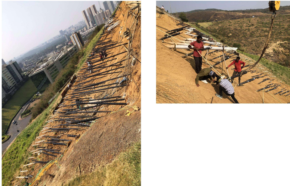
ANCHORING ANCHOR BARS AND FIXING OF M.S PIPE ENCASING
