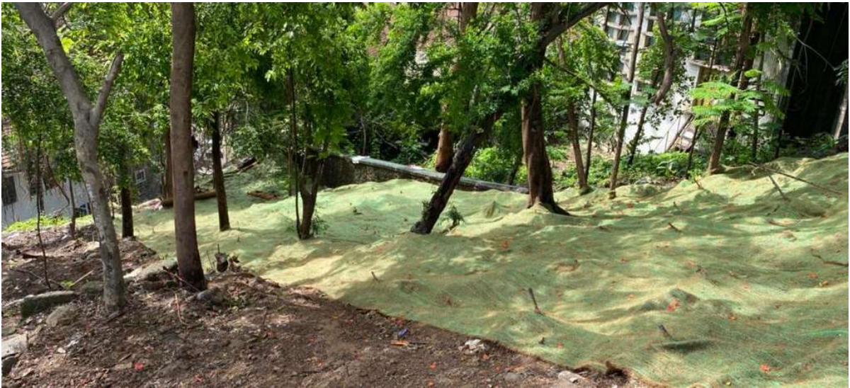
Site Photograph: Installing Erosion Control Mat
