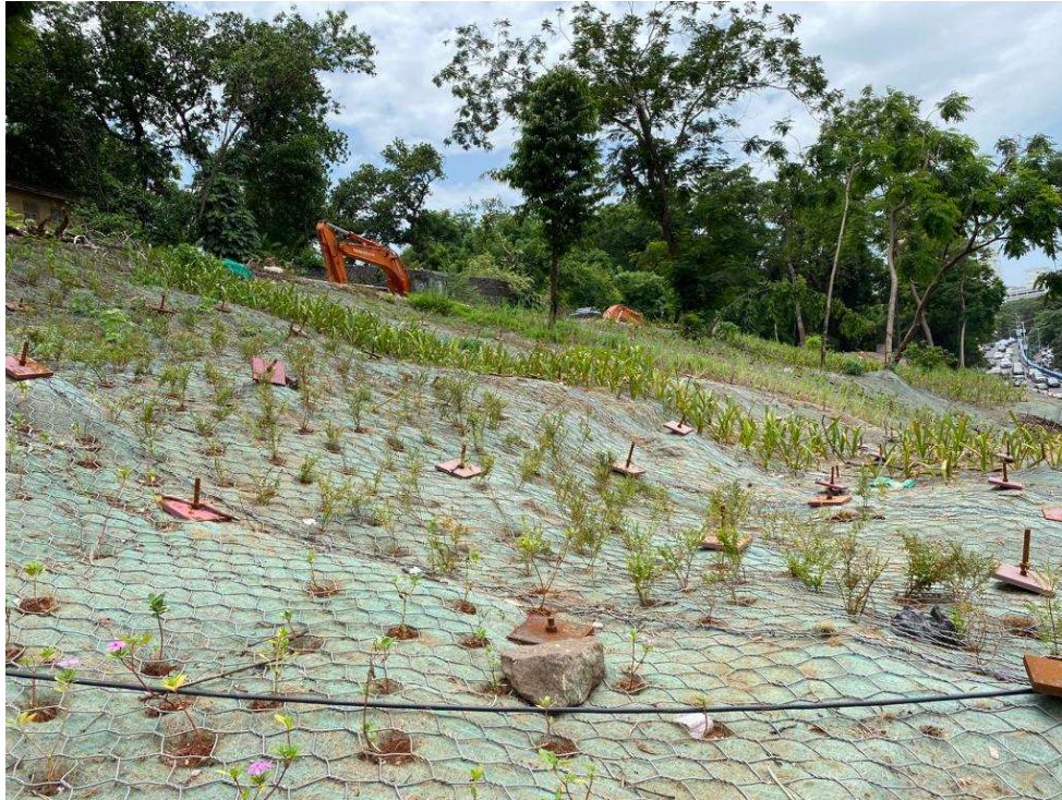
Site Photograph: Plantation of Vegetation on Slope
