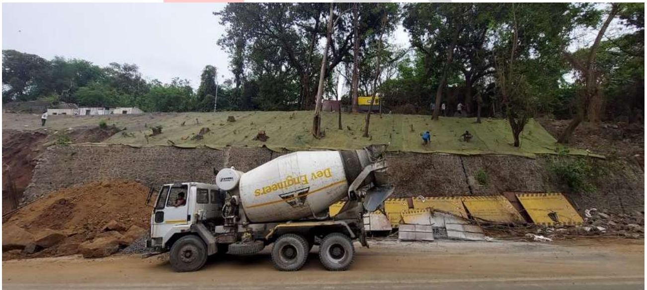
Site Photograph after Completion of work.
