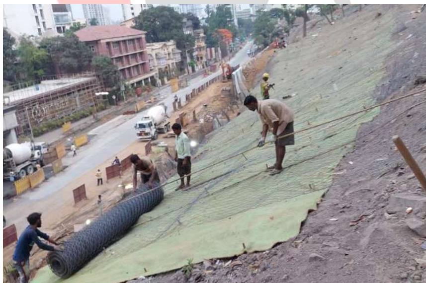
Site Photograph: Installing DT Netting Over Erosion Control Mat
