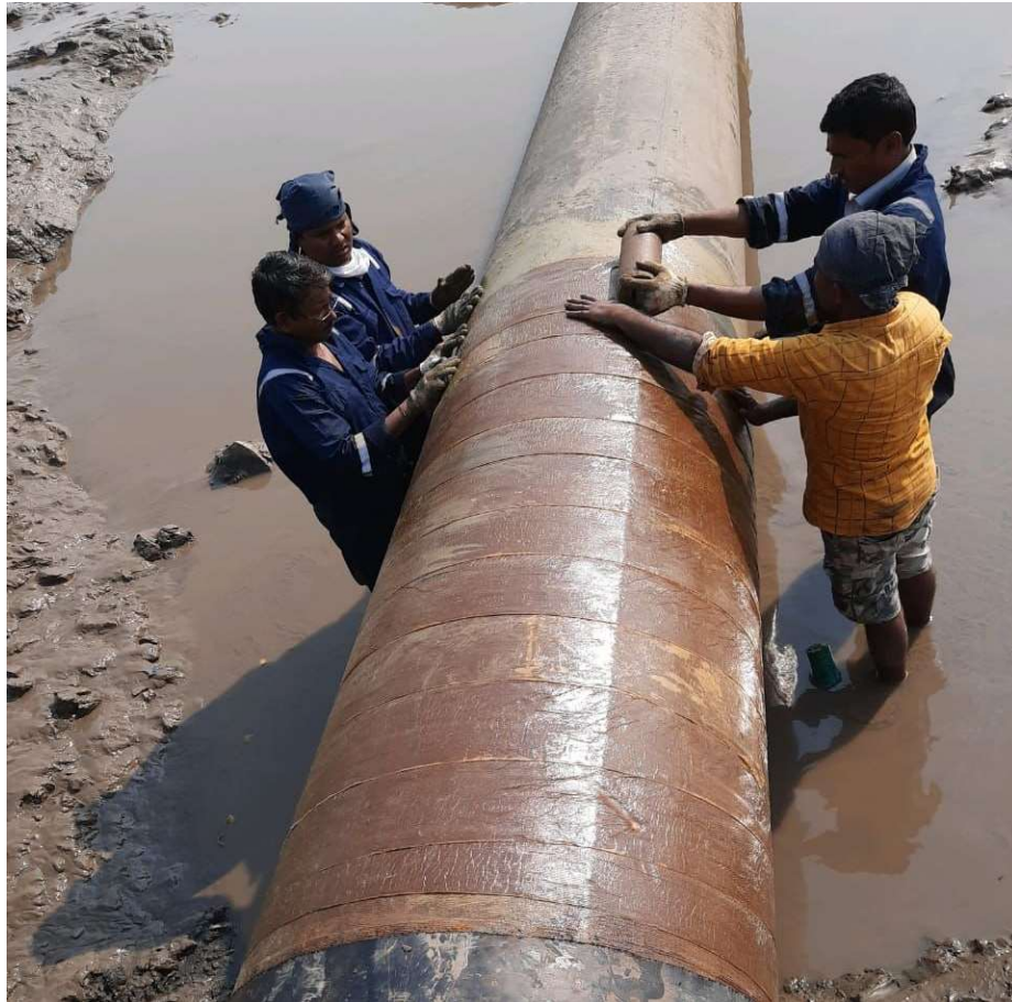
Pipeline Coating Repair Works
